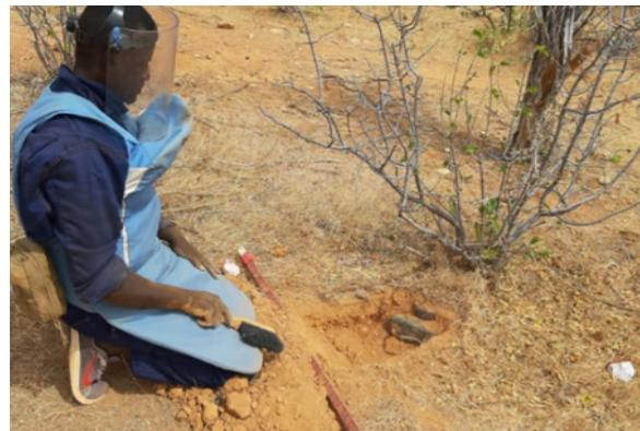
Fig 13: MDT deminer excavating an AT
